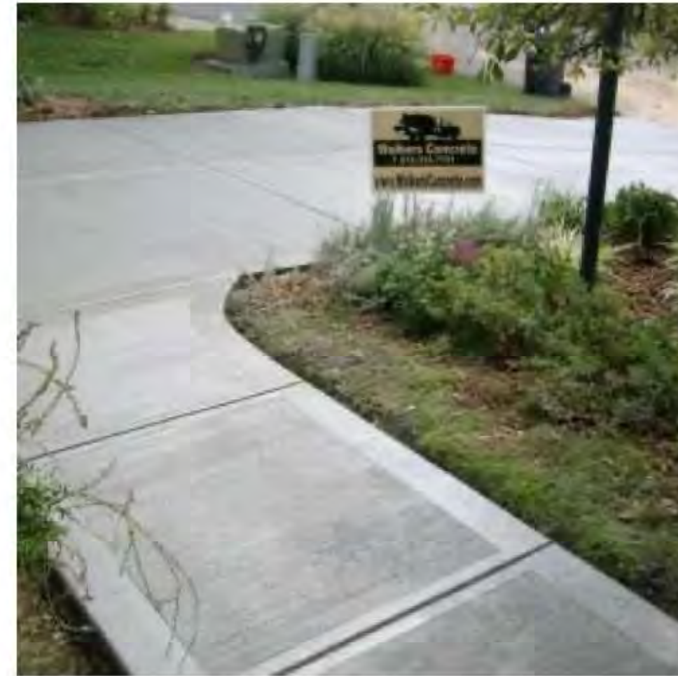
CIP CONCRETE PAVING
