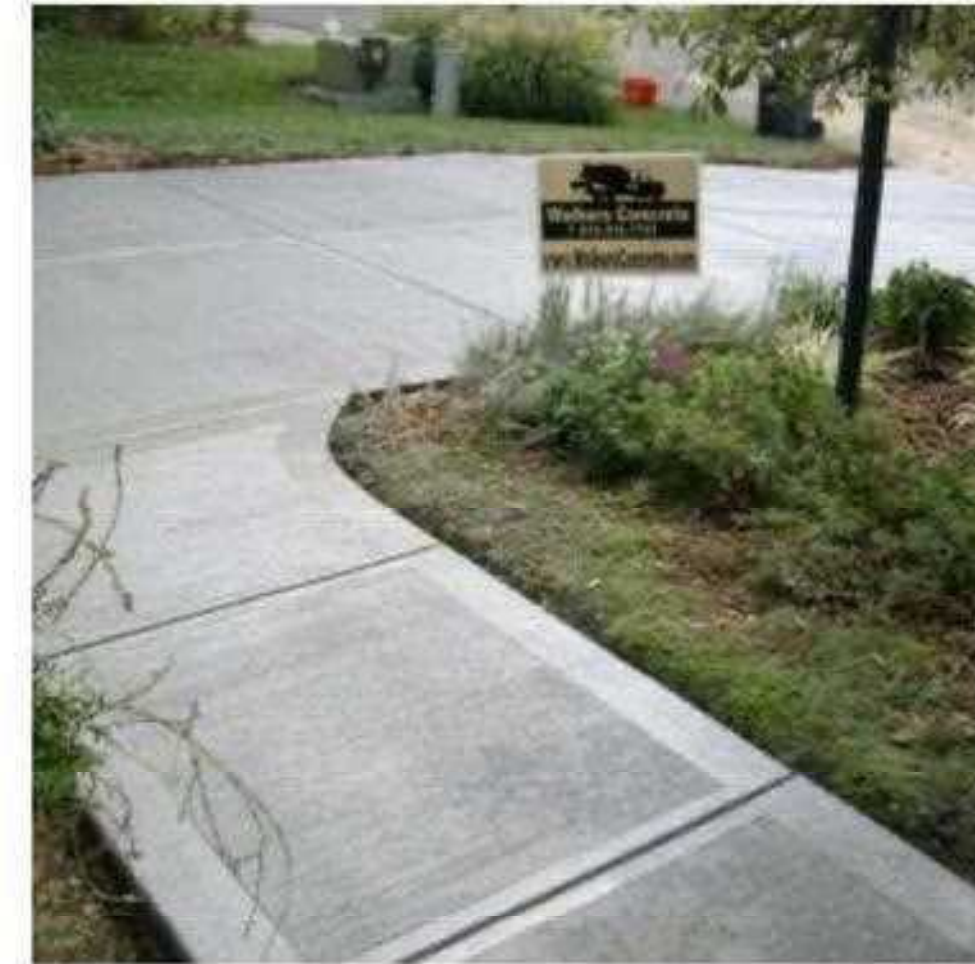
CIP CONCRETE PAVING
