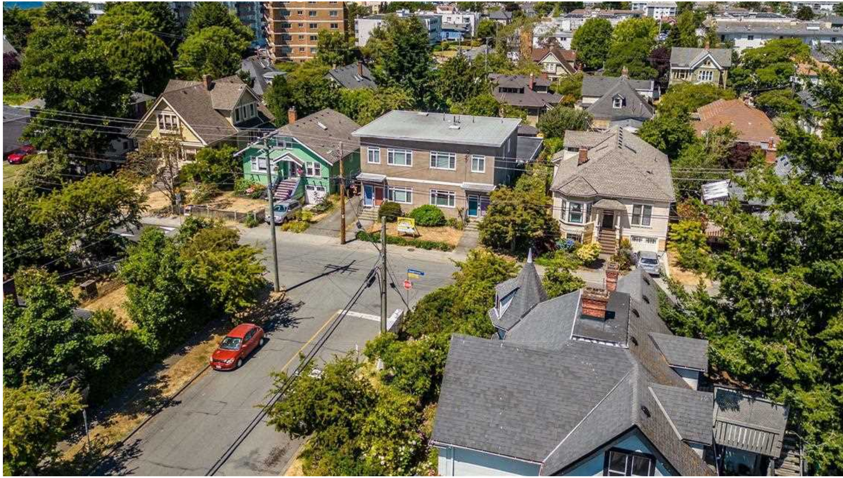
1 Existing Building, 50 Government
